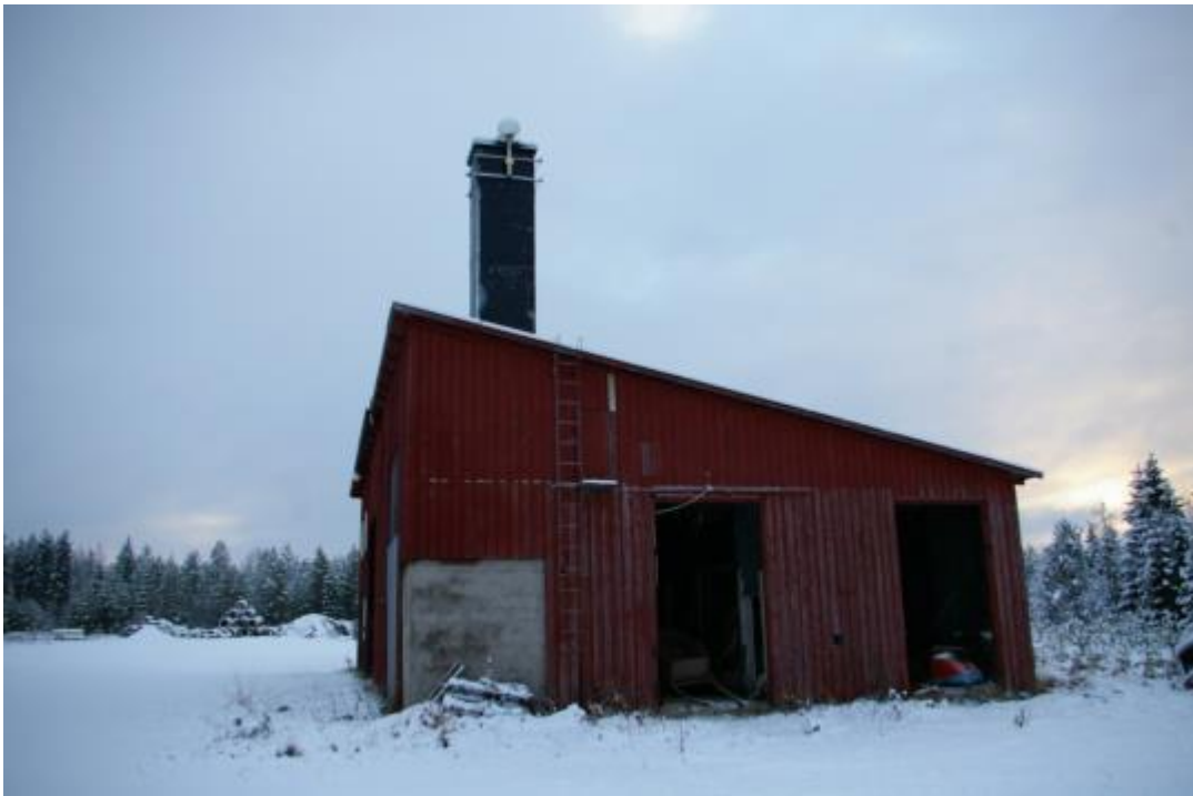
Photo for the mounted antenna of station Botsmark
