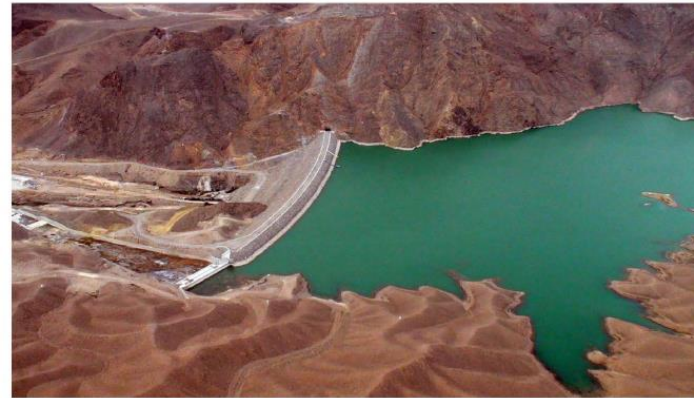
Damghan reservoir rockfill dam
