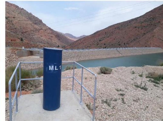
Mojen reservoir rockfill dam
