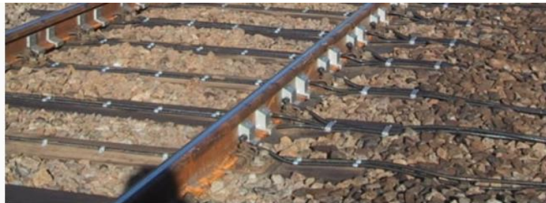
Sensor-based derailment detection system "Argos Derail"
